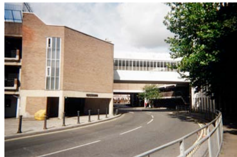
Bridge to car park over Old Greyfriar Street
